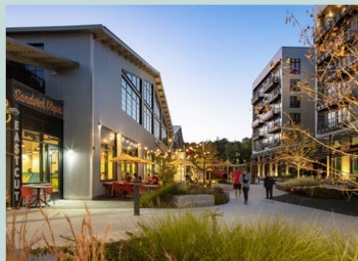
RALEIGH IRON WORKS / Raleigh, NC
