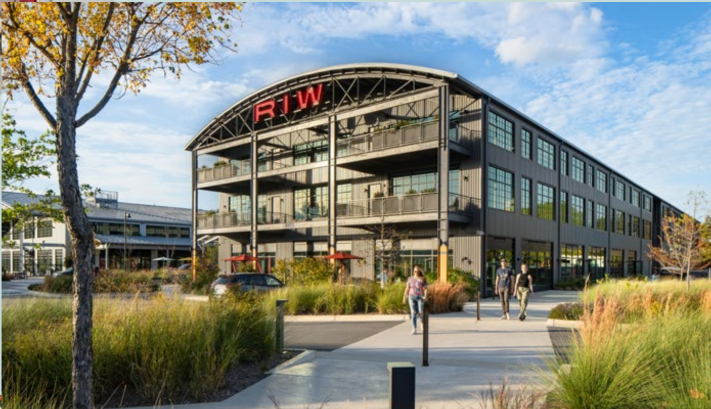
RALEIGH IRON WORKS / Raleigh, NC
